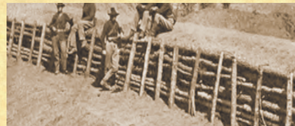
The earthen walls of the fort may have been revetted, or supported with logs, like that pictured above.
