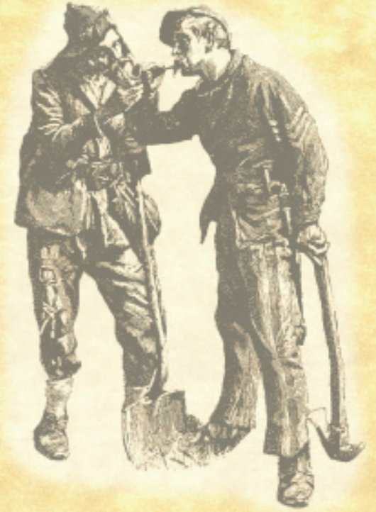
The Civil War fort at Boonesboro was not constructed with machines but by men, using only hand tools. Capt. Brooks' plan specified the exact number of men and tools need to build the fort in the time allotted - 40 men with 10 shovels, 10 axes, 10 picks, one hand saw, one square, one two-inch auger, one adz and two one-inch chisels.
